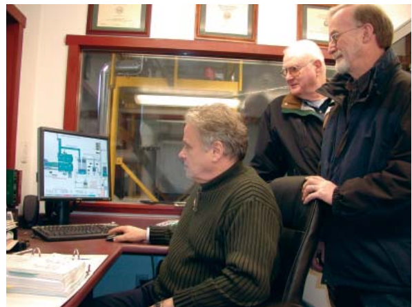
Control Room with Data Acquisition and CEMS system for continuous monitoring
