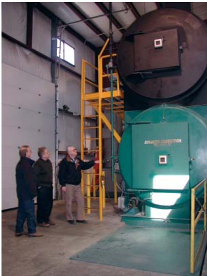
ACS MODEL CA-750MSW with Auto Ash Removal and Feed System
